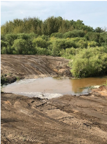
Before (right) and after (above, before seeding) of a stream crossing installed to decrease erosion from livestock.
