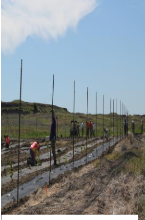
T-posts being installed for the fence
